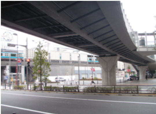
Figure 4 AKIBA pedestrian bridge constructed with HSC ( f'_c = 120 MPa) in Akihabara
