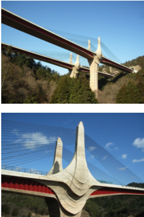
Figure 19 Rittoh Bridge (Extradosed PC bridge with corrugated steel web)
