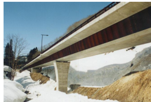
Figure 18 Ginzanmiyuki bridge with corrugated steel web
