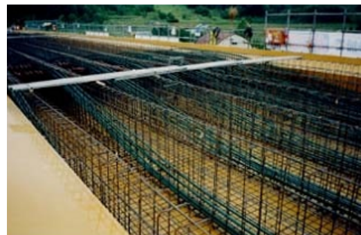
Figure 3 Use of pre-grouted prestressing strand for main tendons
