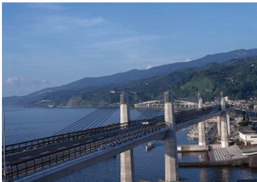
Figure 15 Odawara Blue Way bridge
