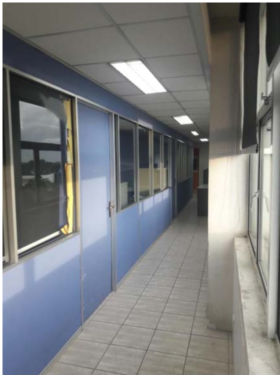
Figure 4: Entrance of cabin 1
