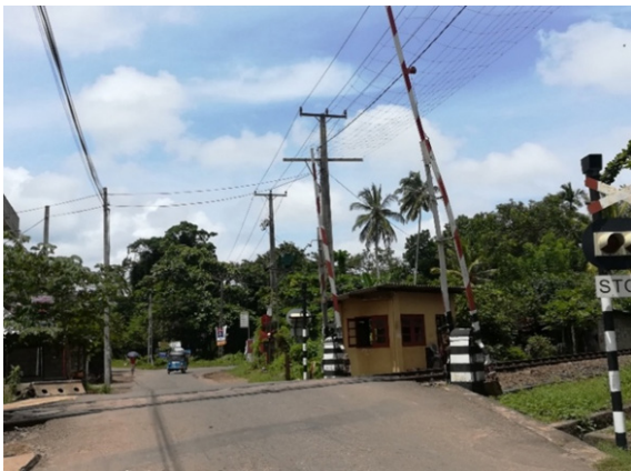
Figure 4. Barrier Equipped Mechanical Level Crossing in Sri Lanka
