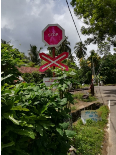
Figure 8. Safety Signs fixed too close to the Level Crossing
