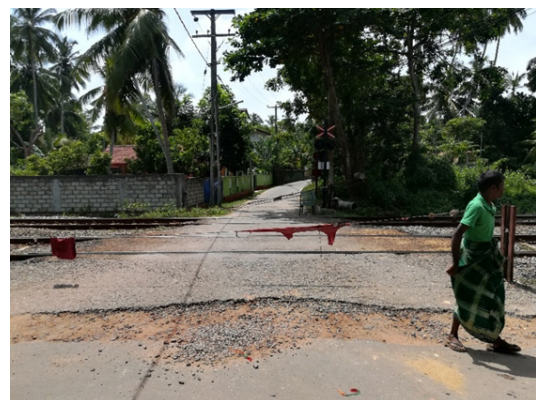
Figure 7. A GI Gate replaced with Rope and Red Cloth
