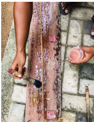
Figure 3- Application of Resin
