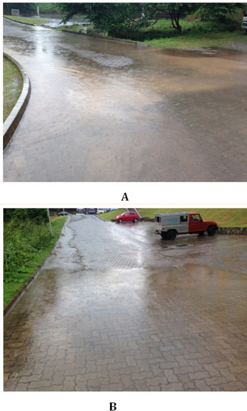
Figure 1: Water pooling in front of Faculty of Engineering due to a small rainfall [2].
